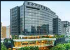
Sofitel Extension, Mumbai Maharashtra
